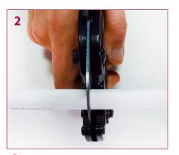
Cut the pipe using a pipe cutter.
