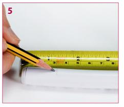
Measure and mark the correct insertion depth on the pipe.
