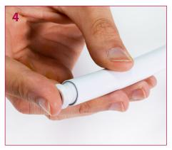
Fit the pipe insert into the pipe.
